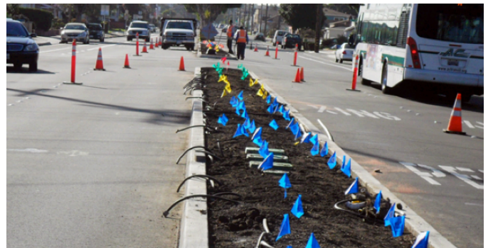
Low flow bubbler style irrigation was used throughout the project. Irrigation in the median is controlled by a 'smart' controller equipped with weather sensors.
